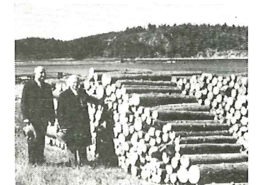
R. A. Hayward, President, and J. Kindleberger, Chairman of the Board, inspect first pulpwood to arrive at Espanola
